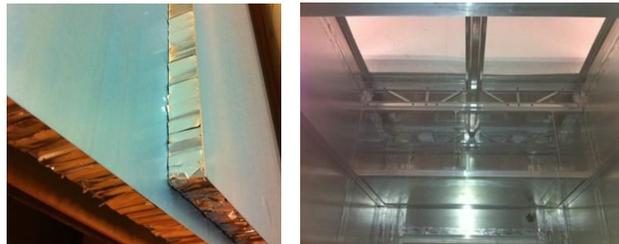
The Clean Room was a modular design using mill finish aluminum extrusions and panels. Basic wall panels consisted of two sheets of aluminum sandwiching an aluminum foil honeycomb. Walls were 2" thick; ceiling panels used the same design but are 1/2" thick. The ceiling consisted of a top plenum cap 10' high which provides the outer air seal and an 8' suspended inner ceiling holding the lights and HEPA filters.
