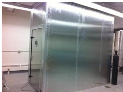
The outer 5'x10' airlock was built as the prototype room to test how well the clean room could be sealed.
