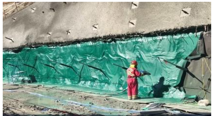
Above: Trans Mountain Burnaby Terminal Right: Application of 150D-FR Spray-Applied Polyurea Site Photos: Courtesy of Layfield Geosynthetics
