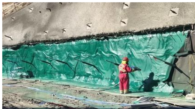
Below: Application of 150D-FR Spray-Applied Polyurea
