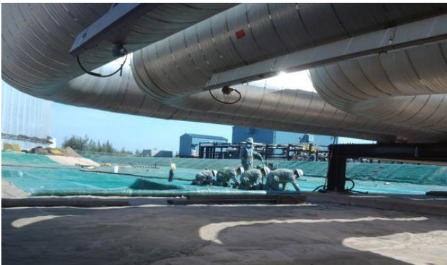
Above: WEC crew installs PRECIDIU TM ECS TM 150D-FR Membrane at Tank Farm in Fort McMurray Photos: Courtesy of Western Engineered Containment
